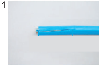
1 Expose inner vinyl sheath.
